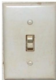
To turn the light on and have it stay on until dawn, flip light switch on, then off for 1 second, then back on. The light will now stay on until dawn or until you turn the light switch off.
